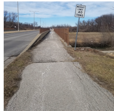
Little Blue Parkway bridge over Little Blue River
